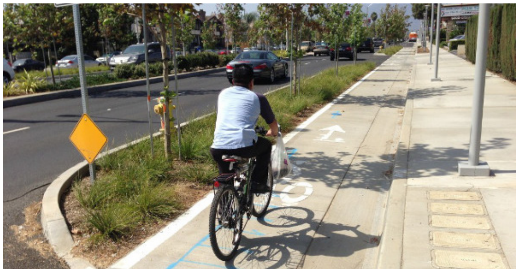
Buffered bike lanes with landscaping and vertical curbs can greatly enhance the safety of the bicyclists while contributing to the streetscape.
