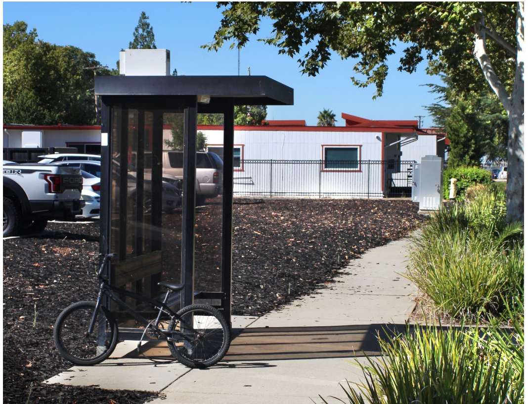
Existing bus shelter on Atlantic Street at Doyle Street.
